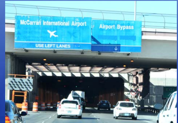
The Airport Connector Tunnel will soon receive new life safety signage.
